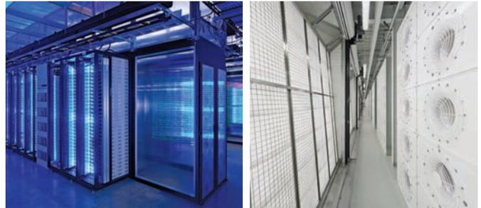
joint venture with Portland, Ore.-based Fortis Construction. Variable-frequency-drive-equipped fans work in concert with onboard server fans to draw air over the server components at the ideal rate.
